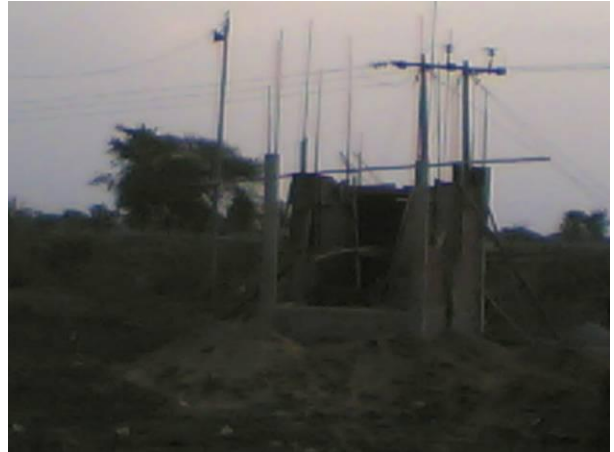
Construction of watch tower under progress
