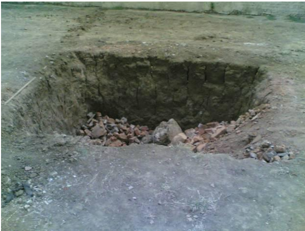
Water harvesting pond
