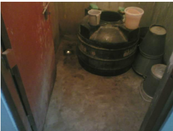
Bathroom inside staff quarter
