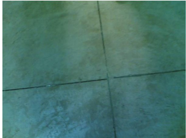
Flooring of the Staff Quarter
