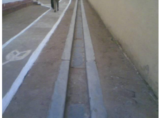
drainage system constructed under scheme
