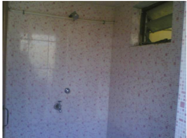
Bathroom inside staff quarter
