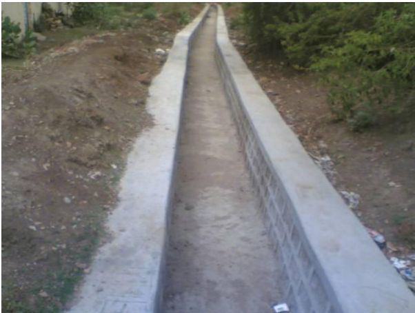
Drainage system built under scheme
