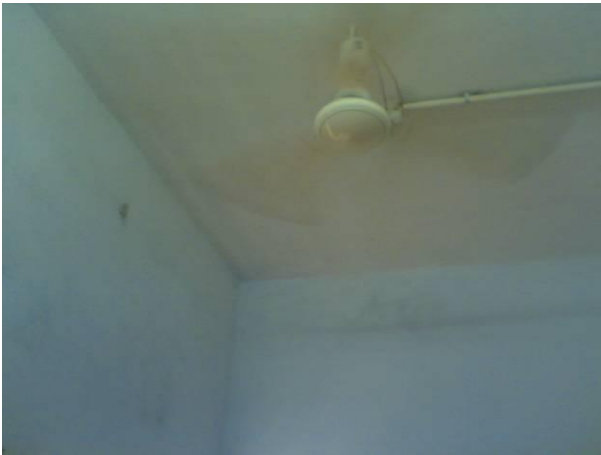
Roof of staff quarter
