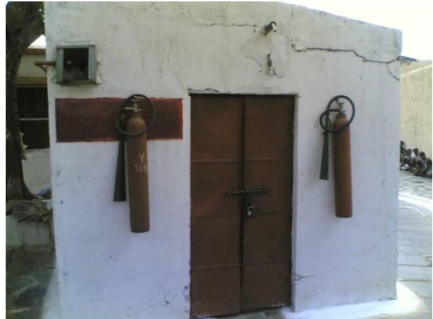
Fire Extinguishers outside the Kitchen
