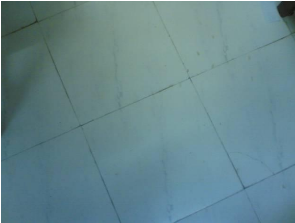
Flooring of administrative office
