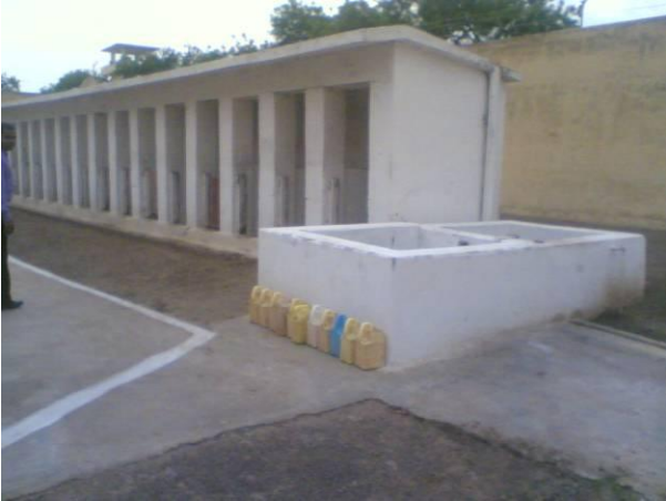
Day toilets and water tank
