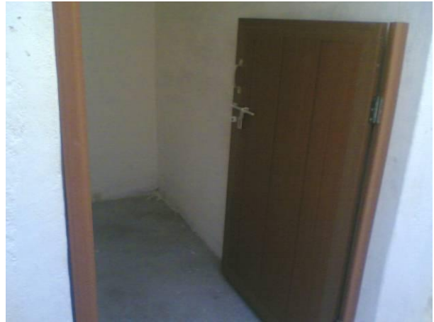
Bathrooms constructed under scheme
