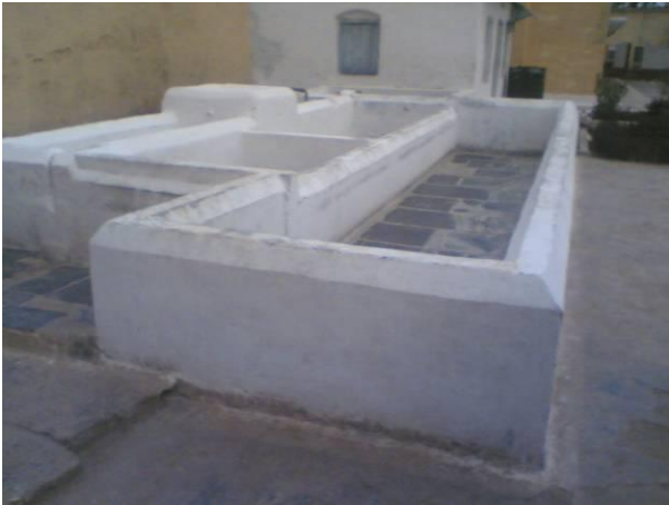
Water tank inside the prison
