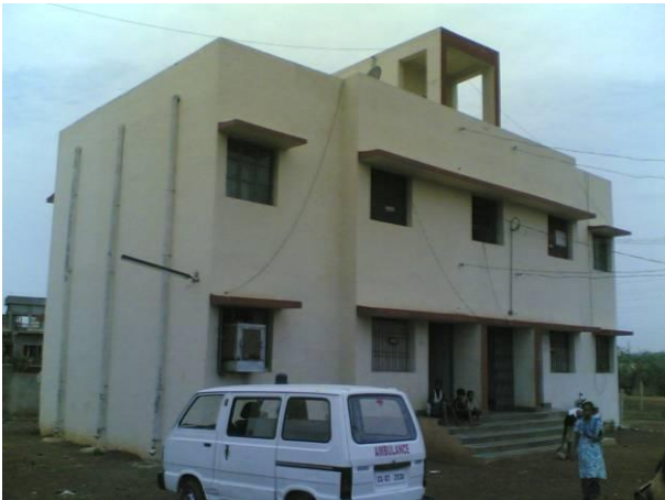
Staff Quarters constructed under the scheme
