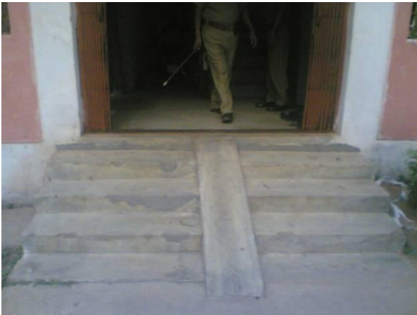
Entrance of staff quarter building
