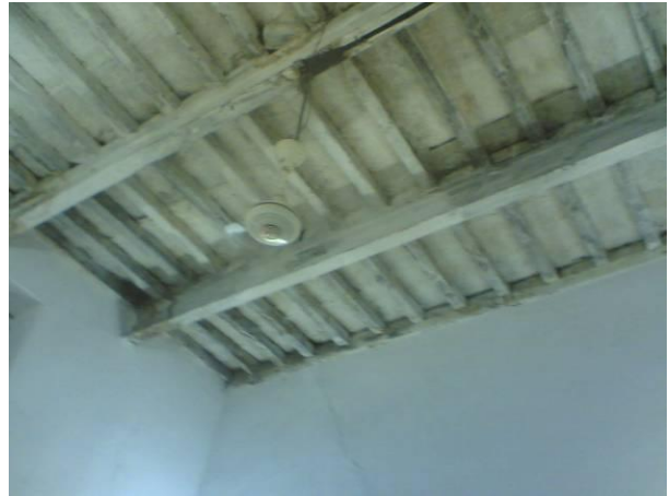
Roof of administrative office
