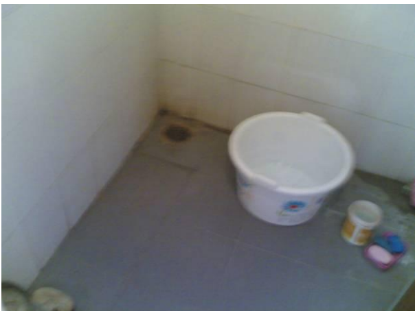
Bathroom inside the Staff Quarter
