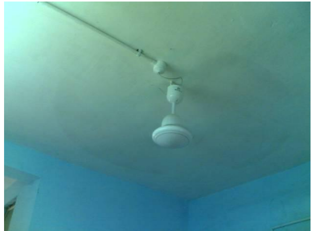
Roof of the Staff Quarter
