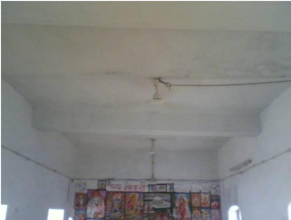
Roof of the prisoner barrack
