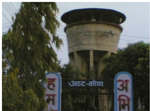
Watch Tower inside the prison
