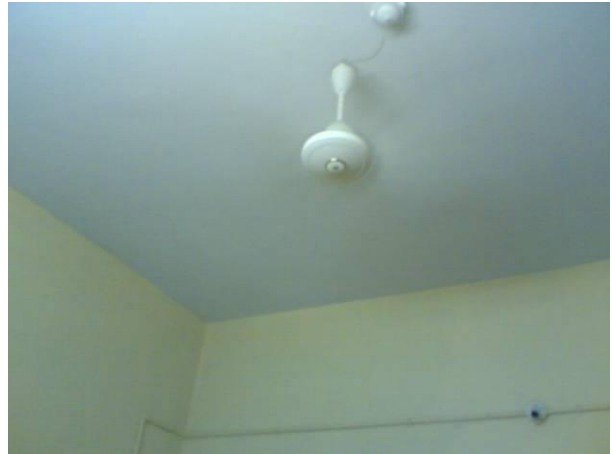
Roof of the staff quarter
