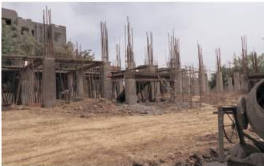
Construction of K9 Handler's Hostel
