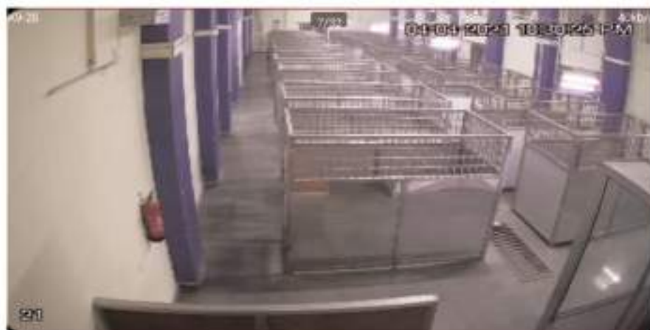
CCTV view of Canine Shed –SS Steel Kennels lined within.
