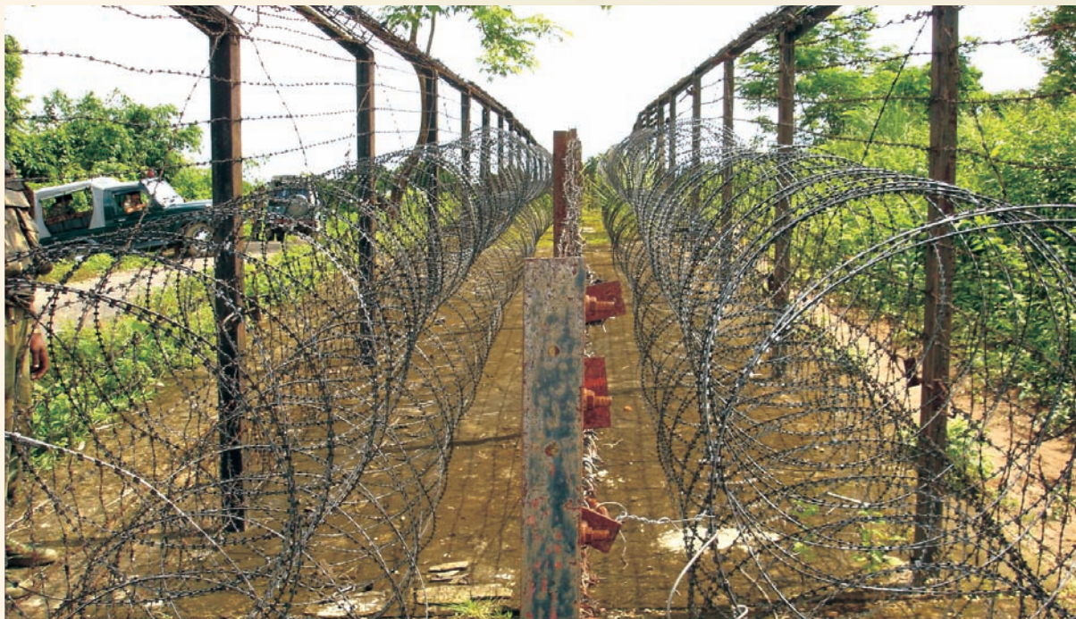
Fencing constructed along Indo-Bangladesh Border
