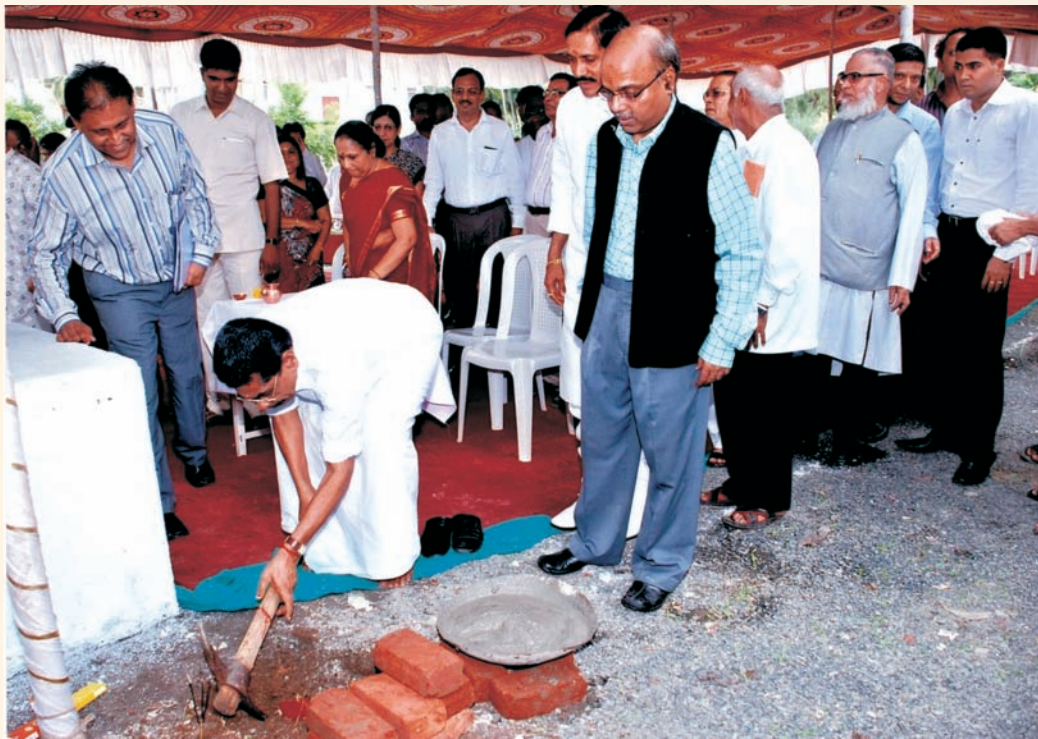
Laying of foundation stone for construction of new OPD Block at Government Hospital, Marwad, Daman by Shri Mullappally Ramachandran, Union Minister of State for Home Affairs
