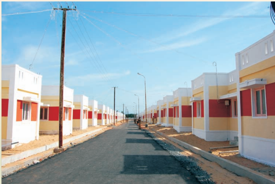
Tenements at Narambai Village, Puducherry
