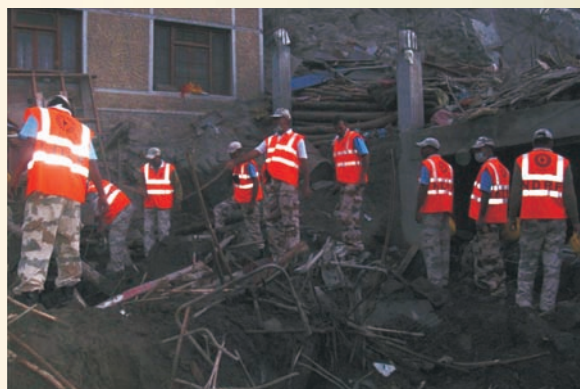
NDRF personnel clearing the debris in Leh- August, 2010.
