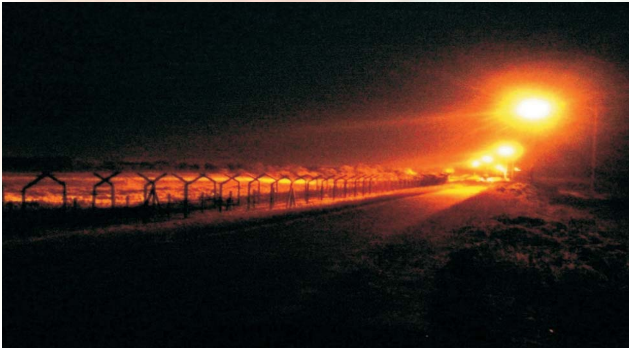
Flood Lighting along the Indo-Bangladesh Border in West Bengal
