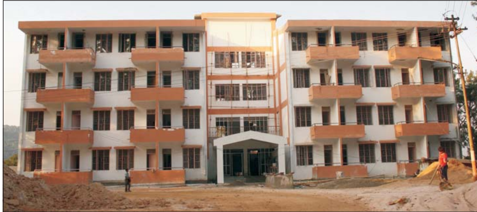
Cadets' Mess under construction
