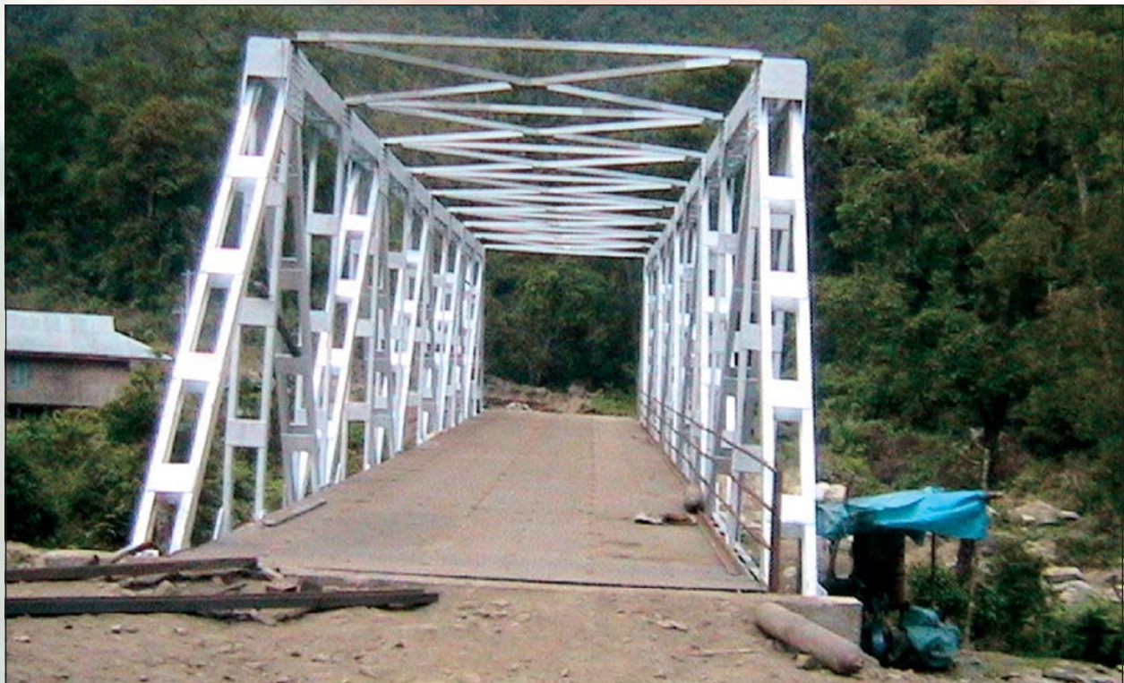
Bridge constructed under BADP over river at Khazlang, Nafra Block of District West Kameng , Arunachal Pradesh
