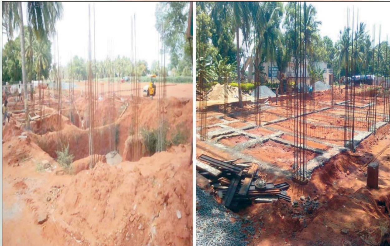
Sewerage Treatment Plant at Lawspet (Under Construction)
