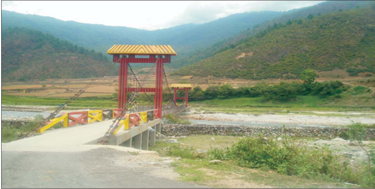
Foot suspension bridge constructed at Bomdila, District West Kameng, Block Nafra, under the BADP over river
