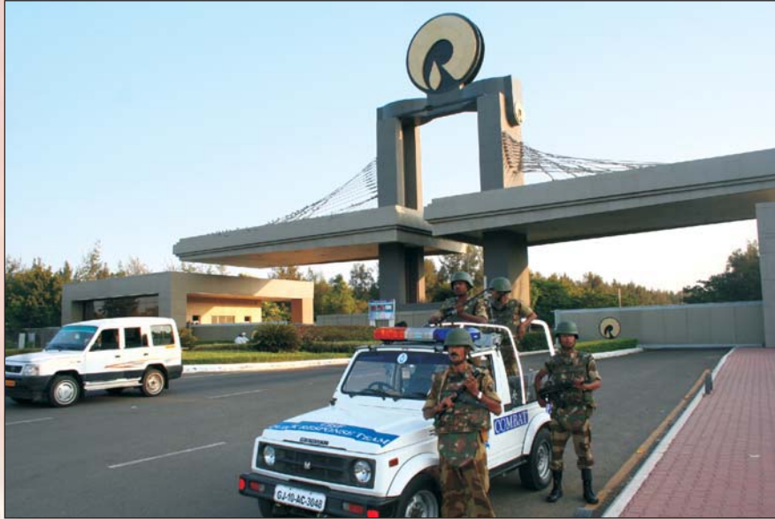
CISF personnel at the entrance of the Reliance Refinery and Petro Chemical Complex, Jamnagar (Gujarat)
