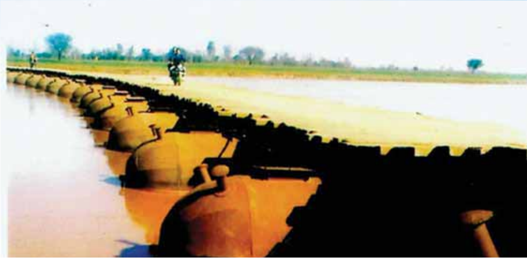
Construction of Pontoon Bridge under the Border Area Development Programme
