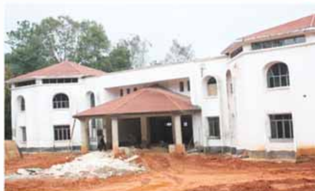
Training Block being constructed
