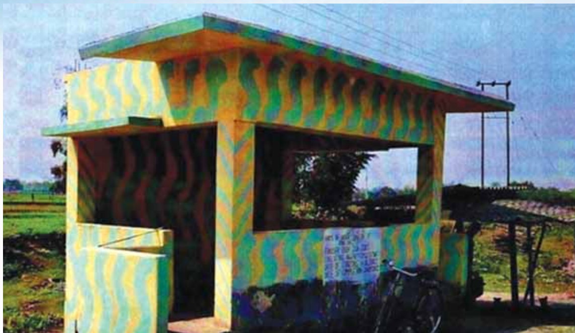
Construction of Rain Shelter on International Land Border under Border Area Development Programme
