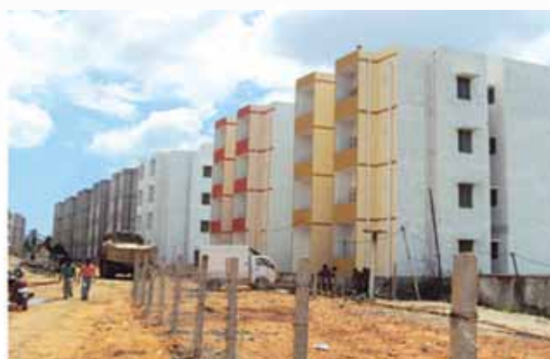
Completed tenement block at Lambert Saravanan Nagar
