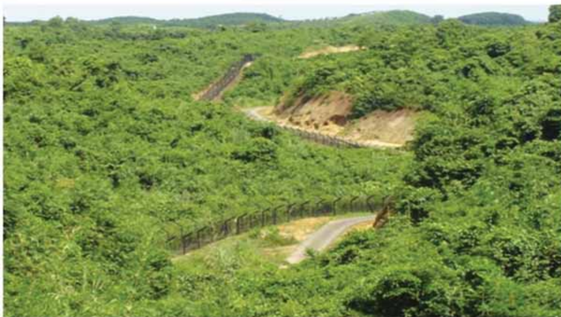
Fencing and road constructed along Indo-Bangladesh Border
