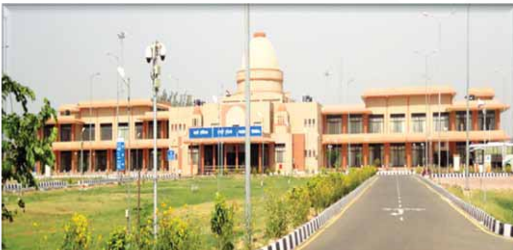
Passenger terminal at Integrated Check Post, Attari.
