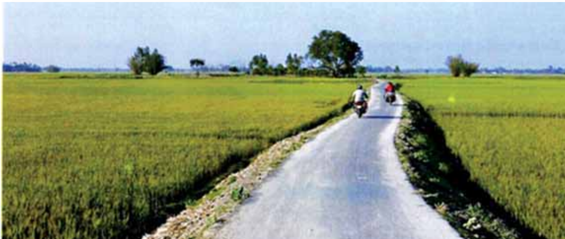
Construction of Road under Border Area Development Programme (BADP)
