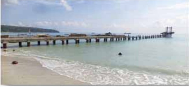
Re-Construction of Jetty at Teresa for berthing of speed boats.
