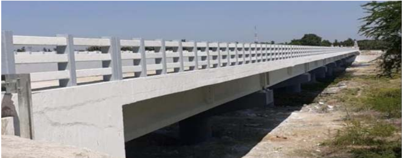
High Level Bridge across Shankaraparani River Thirukanchi, Puducherry
