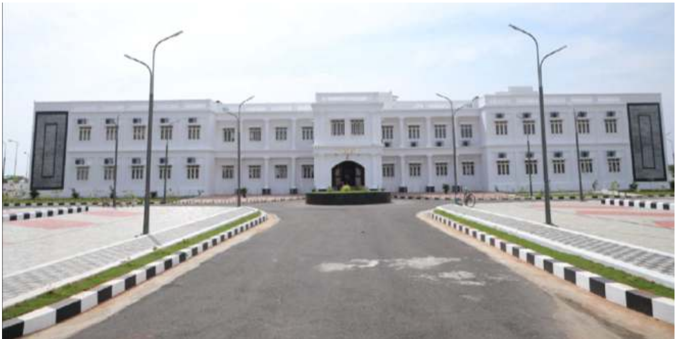
View of combined Court Complex at Keezhaveli in Karaikal
