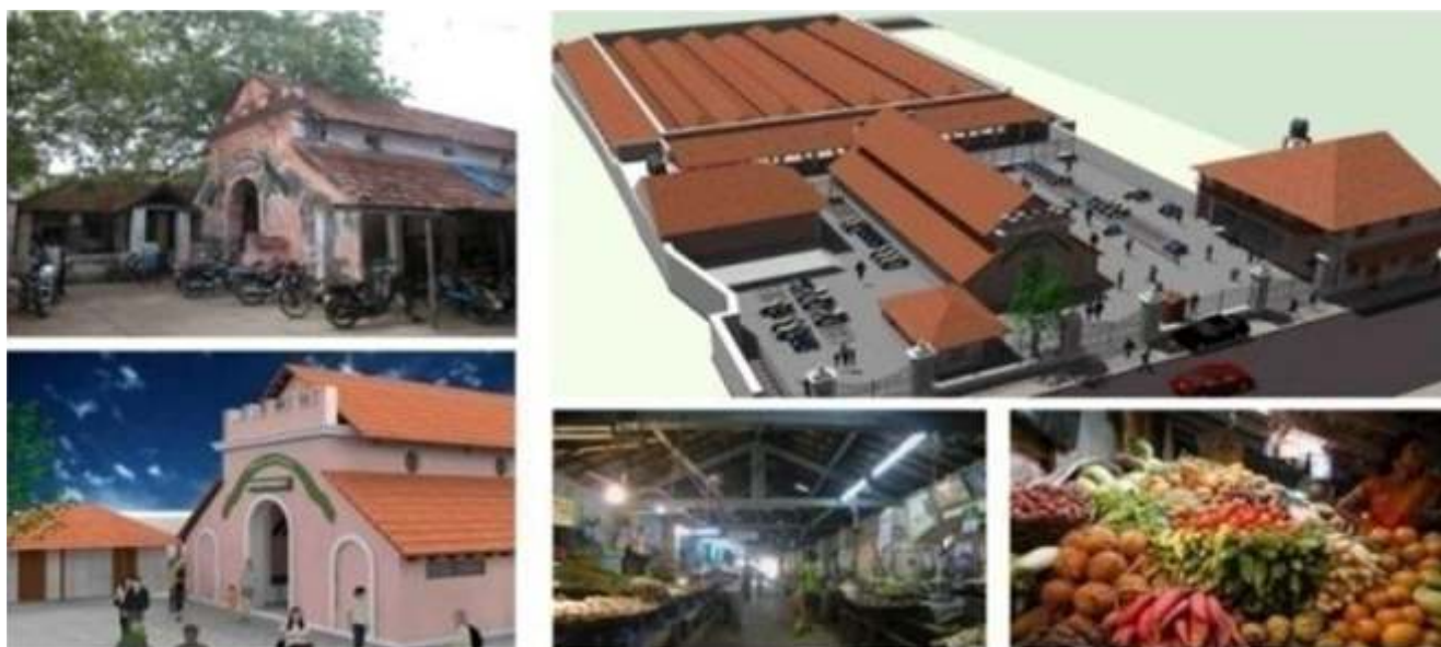
View of Nehru Market at Karaikal after reconstruction
