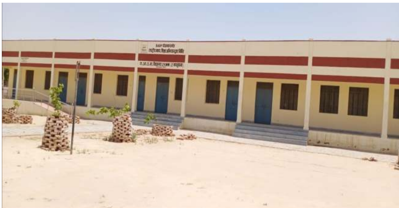
Construction of computer room, art room, science laboratory and library at Government Higher Secondary School, Village: 2 KWM, Block: Khajuwala, District: Bikaner (Rajasthan), Year of Completion: 2019-20.
