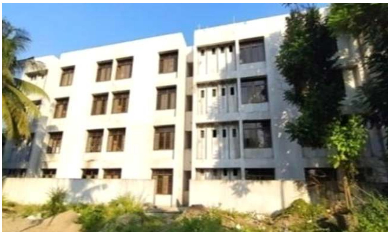
Construction of New School Buildings
