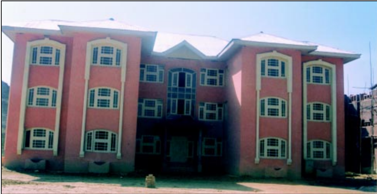
Two bedrooms flats constructed at Budgam
