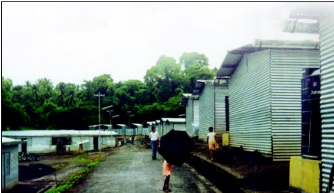
Intermediate shelters at Brichgunj
