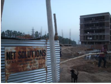
Construction is going on for Net Solutions
