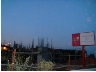
Construction of Five Star Hotel Lalit is going on
