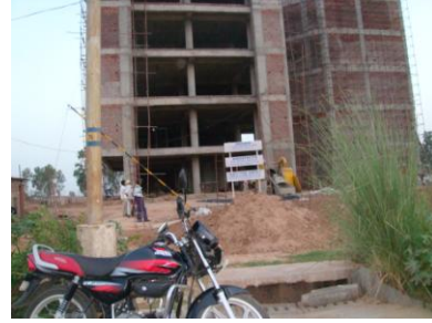
Construction work of Net Solutions
