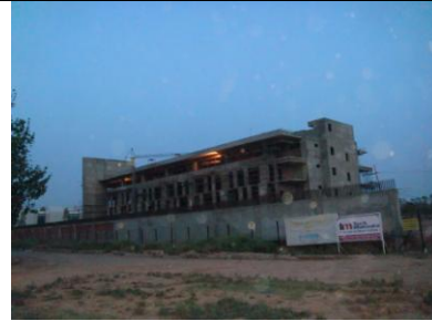
Construction of IT Co. is going on
